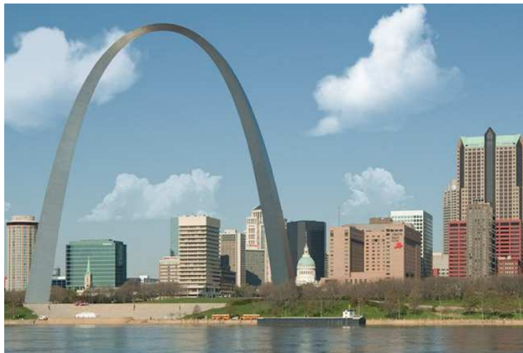
Figure 3: Gateway Arch in St. Louis designed by Eero Saarinen
