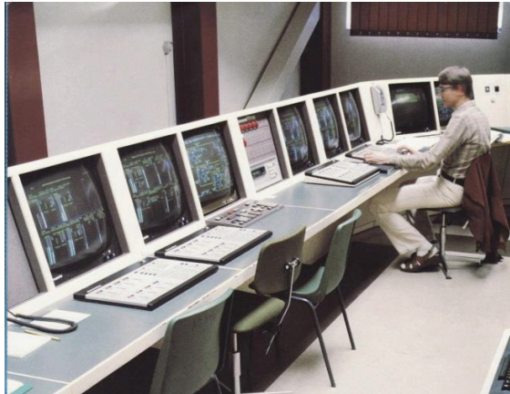
A Damatic control room
